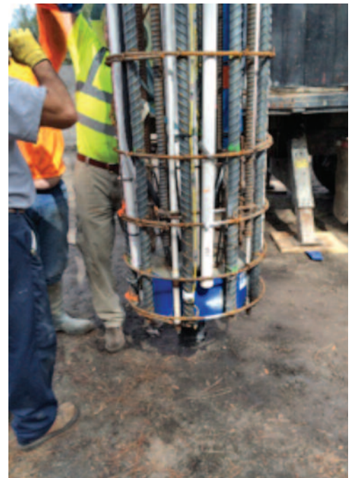
RIM-Cell attached to the bottom of the reinforcement cage.
