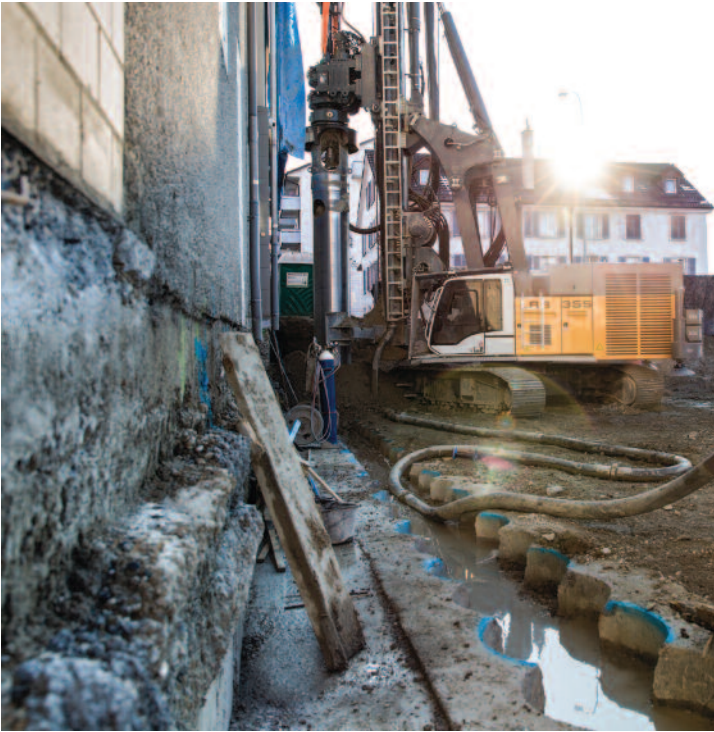
A LRB 355, the newest piling and drilling rig from Liebherr, in operation for the construction company Hilti & Jehle.
